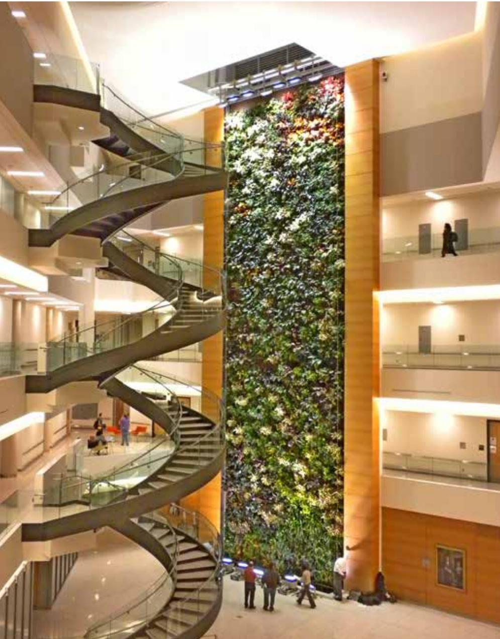
The 80-foot tall biofilter in Drexel University's Papadakis Integrated Sciences building in Philadelphia can purify 15 cubic metres of air per second. *Photo courtesy Nedlaw.*
