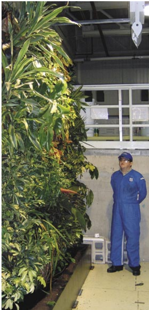
Noel Butler looks up at the living wall in South Paint that has greatly reduced odours for Team Members working in that area. Above, the scale of the installation is clearly illustrated.
